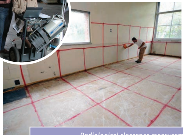
Radiological clearance measurements
