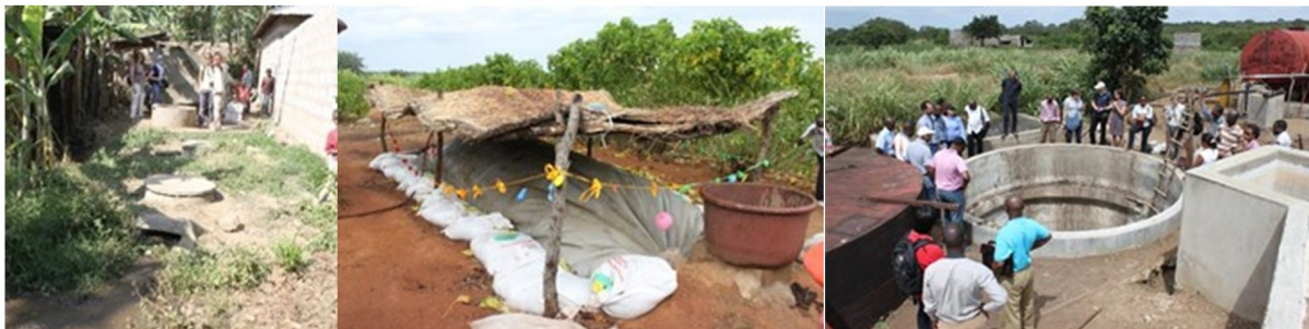
Figure 57: Digester types for household biogas systems in Africa: Fixed Dome Type (underground; Tanzania), Floating Gas Holder Type (underground; Mozambique), Plastic Tunnel Type (aboveground; Mali), source: Dominik Rutz, WIP.
