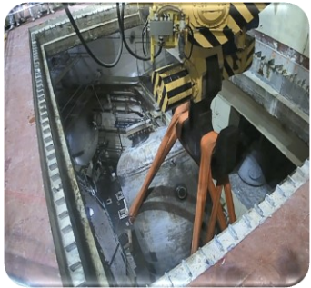
Adjustment of inspection openings above the SGs to transport openings
