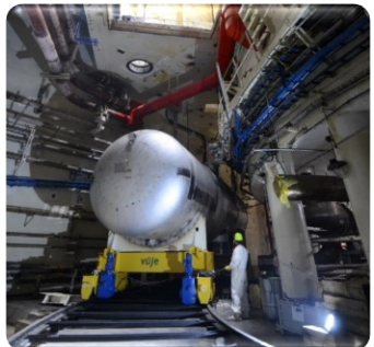
Special railway for transporting the SGs within SG boxes
