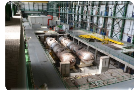
The turbine hall was modified for storage and fragmentation of SGs
