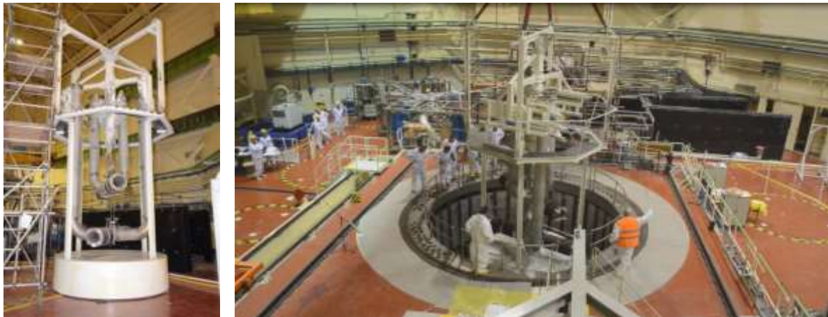
Figure 5: Spider prepared for insertion into the RPV (left) and insertion (right).
