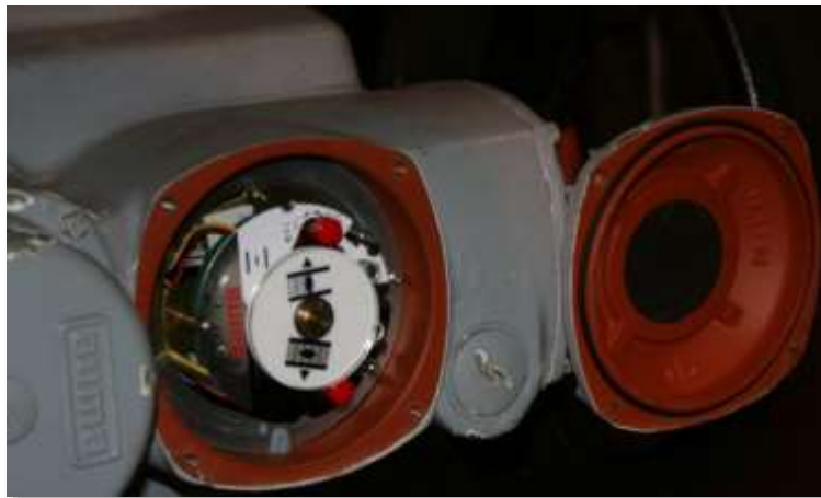
Figure 8. Valve servo actuator with open lid to access to the inner surface.
