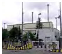
WAK reprocessing plant.
