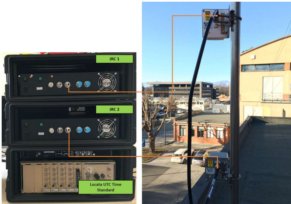
Figure 3-14: Building 72C Installation
