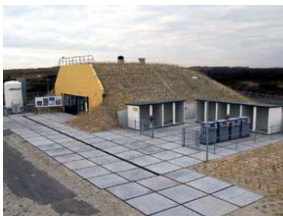
The H 2 tank testing facility
