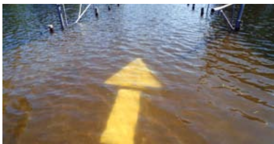
Road flooded by a river
