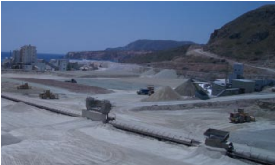
Figure 2-1. Bentonite drying and blending area on the Milos island, Greece.
