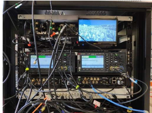
Figure 3.1: Test Rack Hardware Configuration
