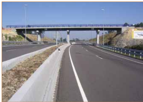
The first European fully vehicular highway carbon fibre composite bridge was installed in Spain
