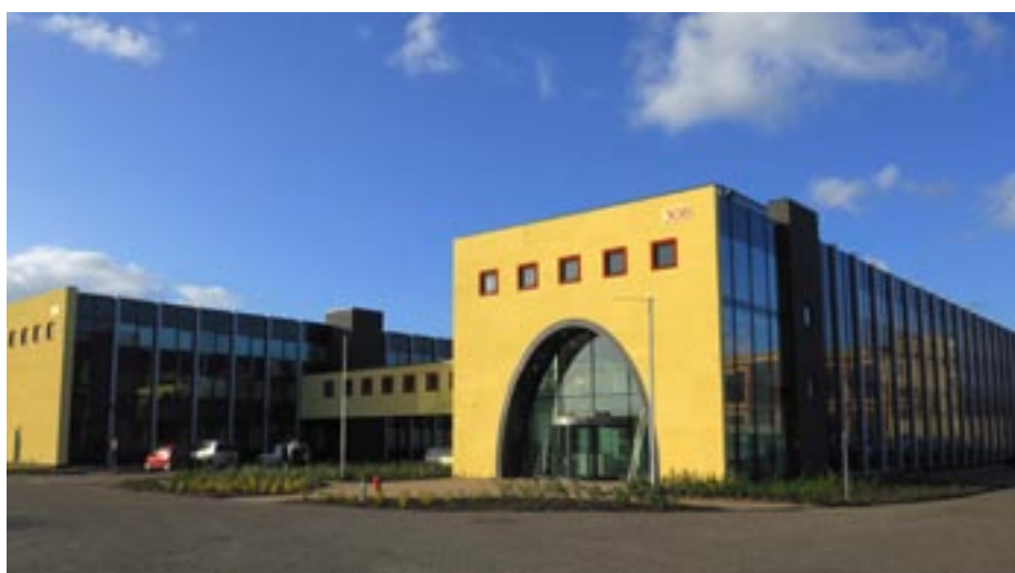
Modern energy-efficient and user-friendly facilities at JRC-IE
