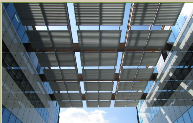
The new and more environmentally-friendly and energy-efficient infrastructure will replace many unsustainable scattered buildings and lead to a 6% energy saving of the JRC site.
