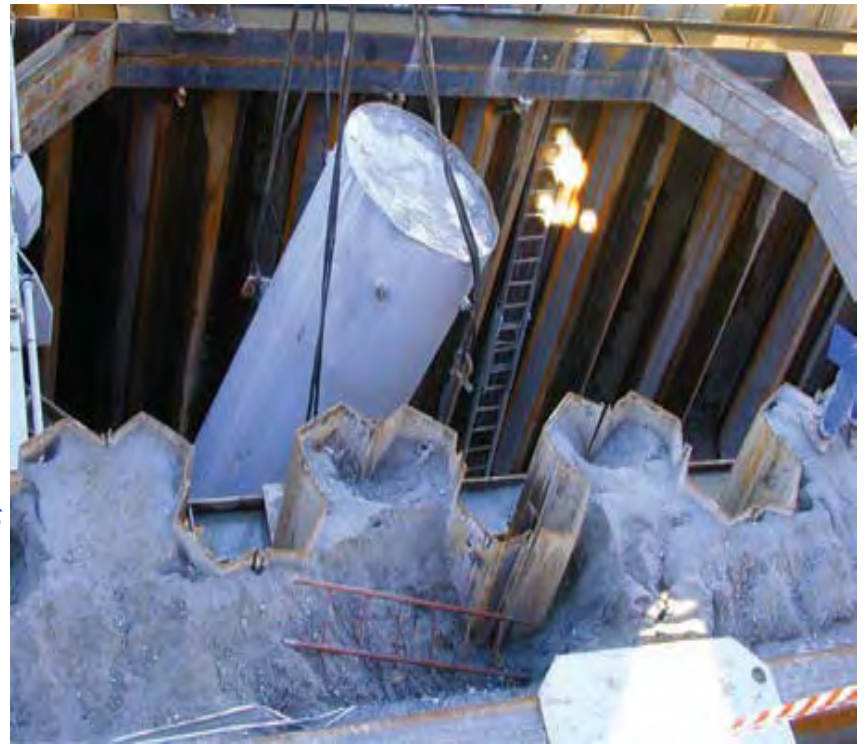
Real scale test of the Roman Pit excavation (Ispra, Italy)
